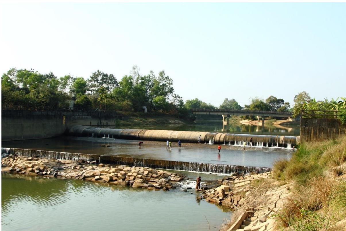
**Fig. 17.** Rubber Dam at Bhuzpur on the upstream of the Halda River.
